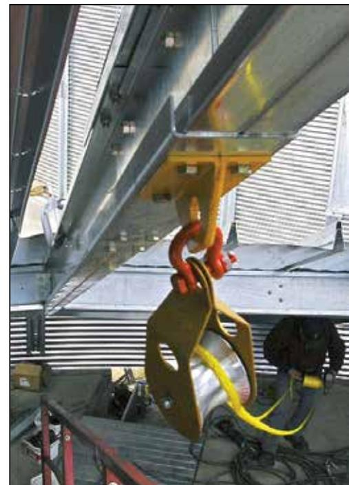
*Steel beam provides a proper anchor point for a lifeline used in grain bin entry.*
