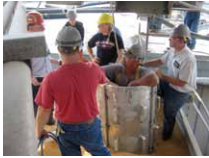
The Andersons cofferdam
