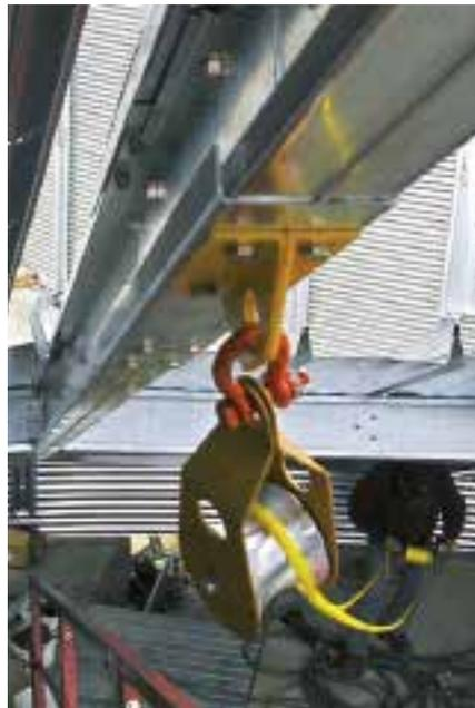
*No practical way exists to address OSHA's bin entry standards without anchor points installed inside grain storage bins.*
